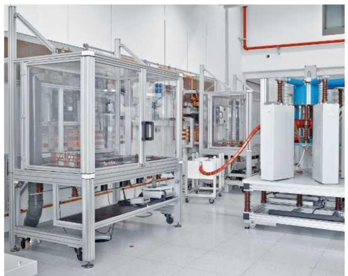
Fig. 25: Testing stations of the high-current testing system
